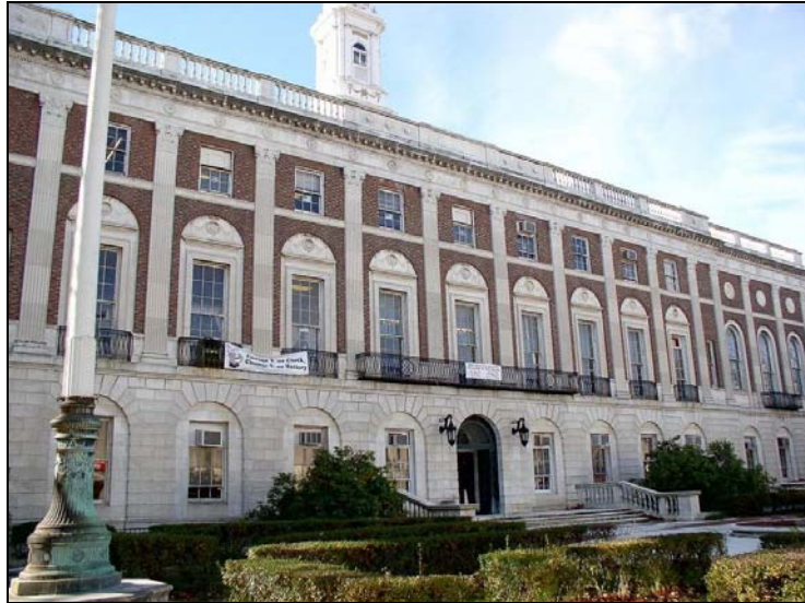
Waterbury City Hall before renovation. Photo: Jerry Dougherty
